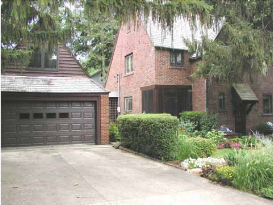
Close-up of garage
