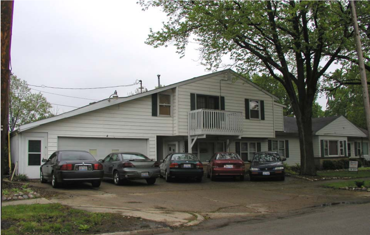
Parking Area as seen from the northwest.
