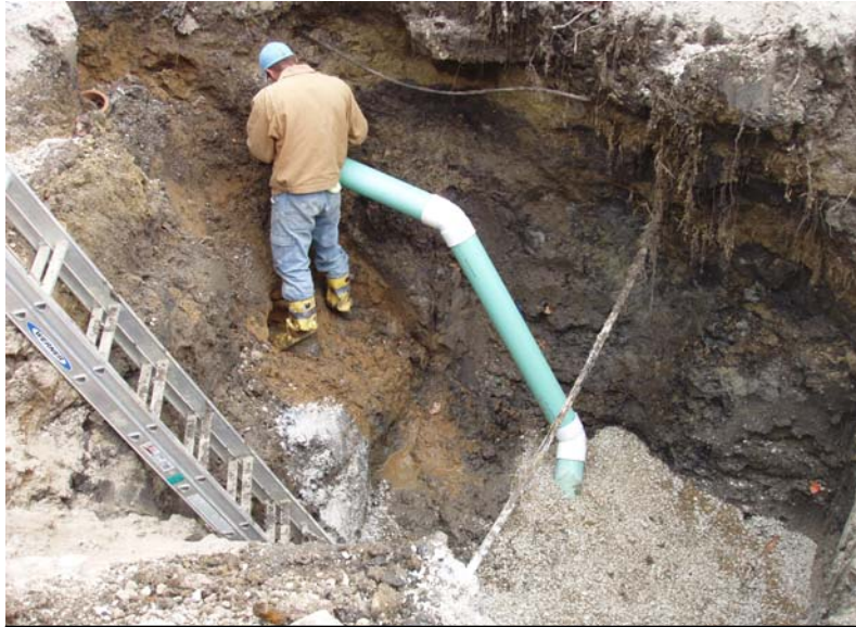
Photo of a typical sanitary sewer service lateral replacement.
