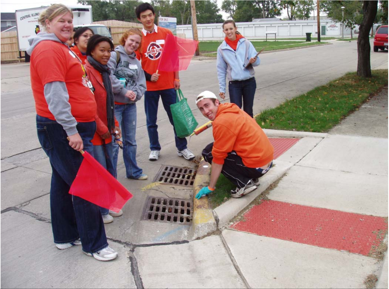
Storm Sewer Inlet Medallion Installation
