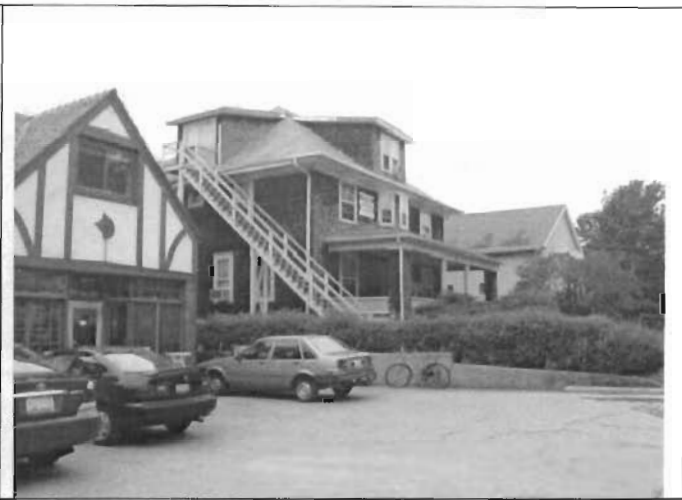
#2 - South west at Café Paradiso parking and retaining wall
