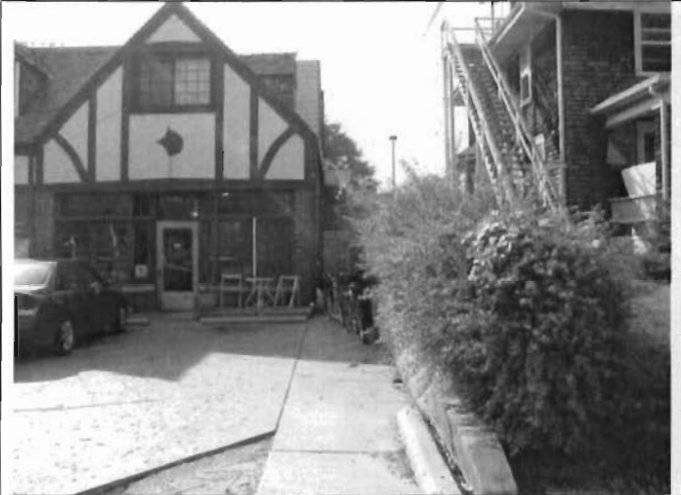
#3 - South down east property line at walk way
