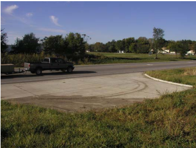
Existing access drive on U.S. Route 150 to serve the development.
