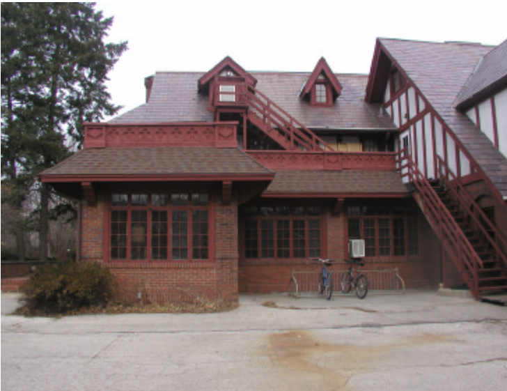
Facing the south side of the Lincoln Green property. (715 W. Michigan)
