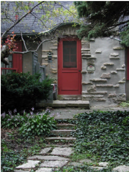
Entryway with stucco and stone chimney
